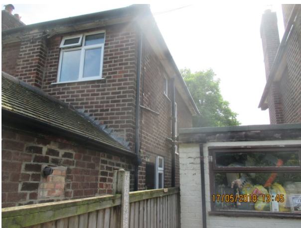
Looking south west towards boundary with no. 7.
